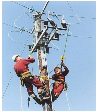
Overhead Line Testing
